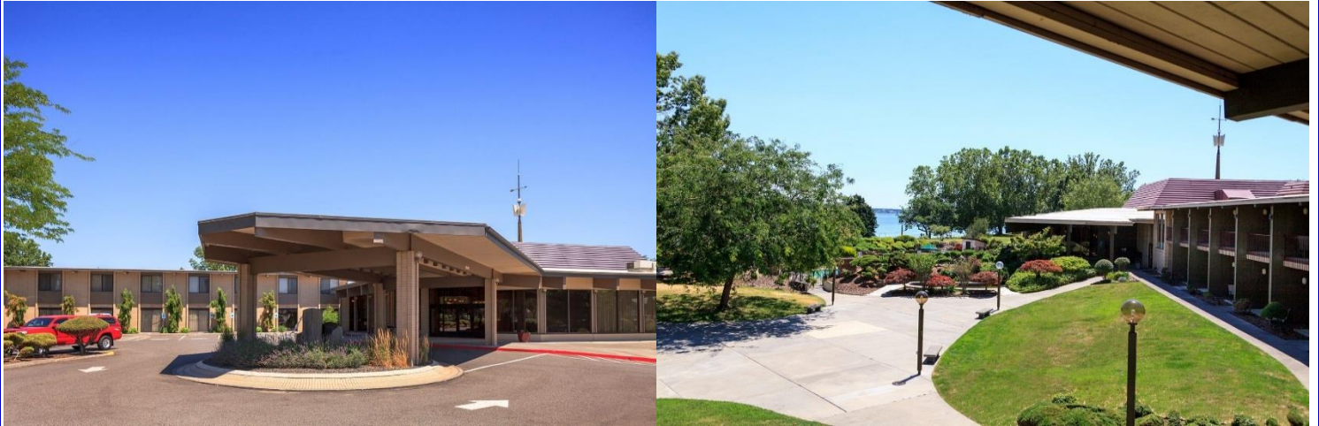
Front and rear pictures of the Red Lion Richland Hanford House Hotel on the bank of the Columbia River in Richland
